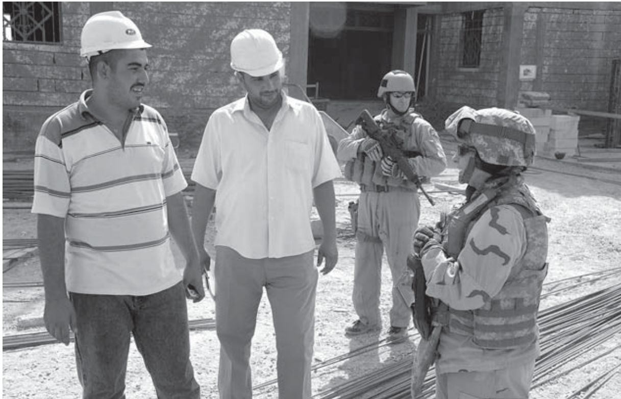
U.S. Navy LCDR Lorraine Luciano, a member of Multi-National Corps-Iraq Staff Judge Advocate office speaks with the on-site foreman about the construction of a new courthouse in the district of At Tannumah in Basra, Iraq, 21 August 2008.
